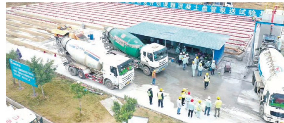
▲ Site of coil pipe test in December 2019
