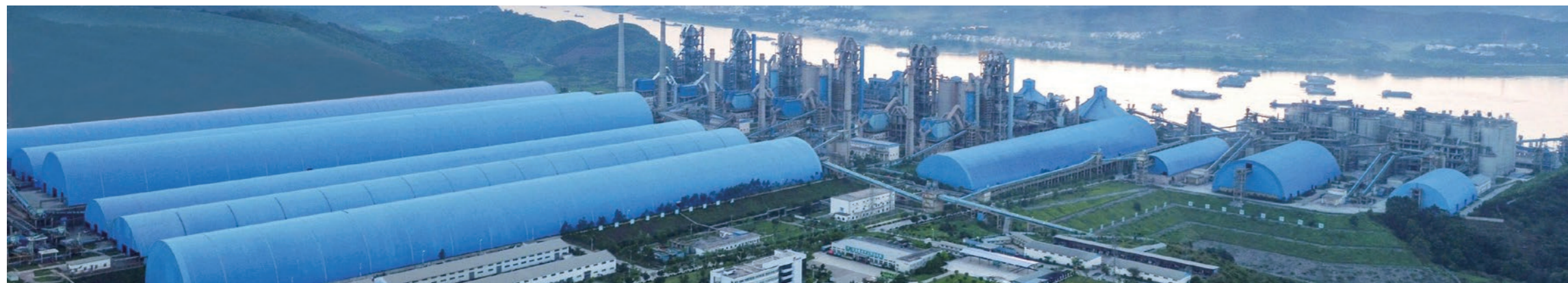
Factory area of China Resources Cement (Fengkai) Limited
