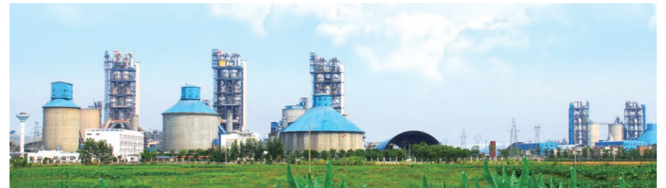
▲ Factory area of China Resources Cement (Pingnan) Limited
