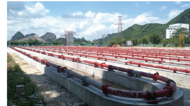
▲ Construction site of "Coil Pipe Test Platform"
