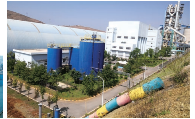
Municipal solid waste co-processing project in Midu, Yunnan completed construction and commenced trial operation
